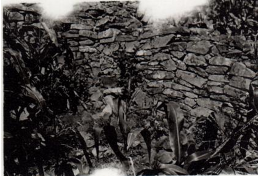
DZATA RUINS – Collapsed walls
