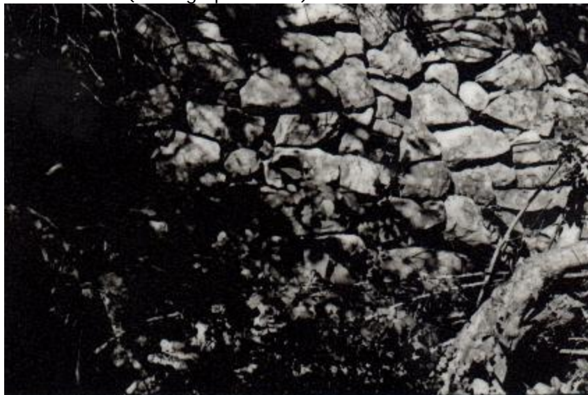
DZATA RUINS – An old wall repaired according to the new style of building (top right corner)
