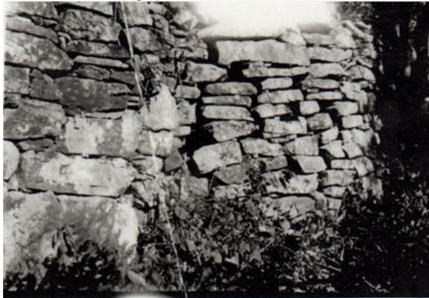
DZATA RUINS – Note stacking on rough foundation stones
