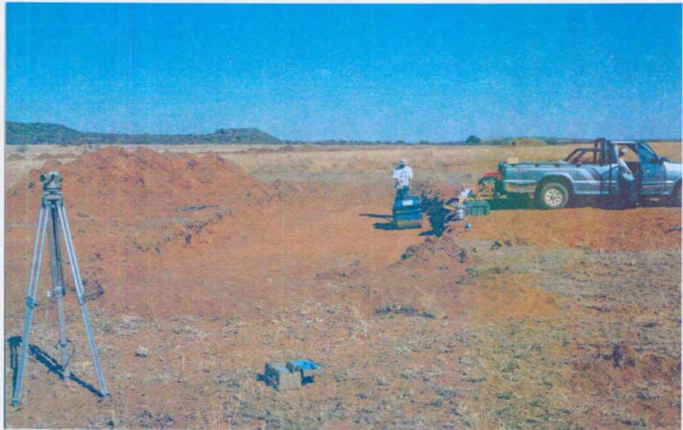
Figure 3.5 Compacting the third layer of backfilled material
