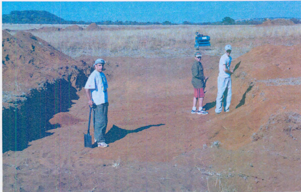
Figure 3.9 Backfilling the second layer by hand
