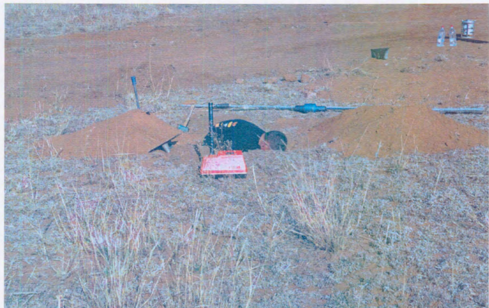
Figure 3.25 Digging the hole for in situ density and DCP measurements
