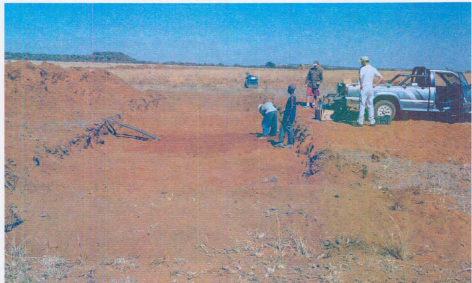
Figure 3.10 Leveling the third layer
