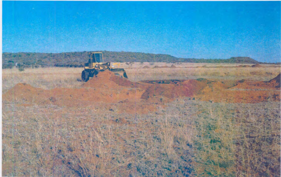
Figure 3.11 Backfilling the last layer using an excavator
