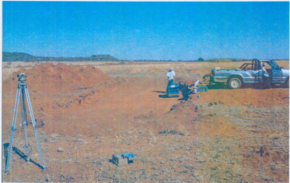
Figure 3.5 Compacting the third layer of backfilled material
