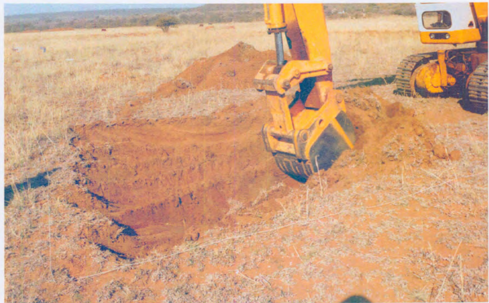
Figure 3.2 Test 2 and 3 excavation close up
