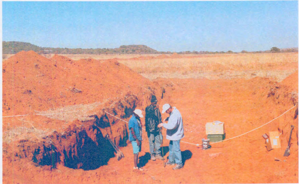
Figure 3.7 DCP testing on a loose first layer
