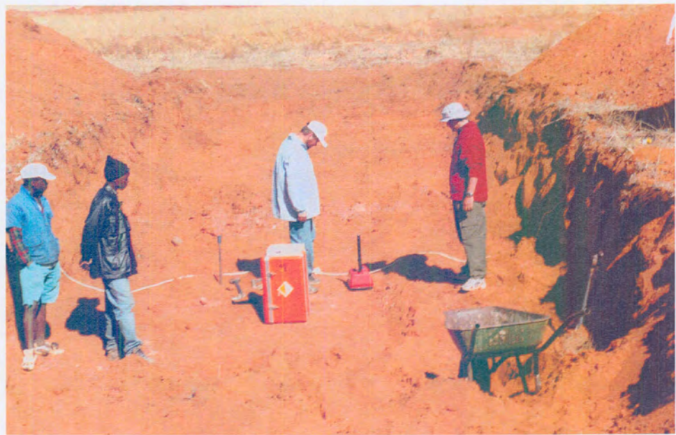
Figure 3.8 Density testing on a loose first layer
