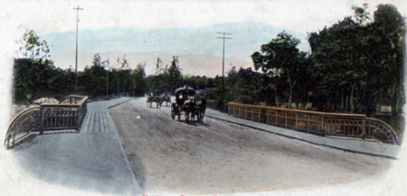
VICTORIA BRIDGE, PRETORIA.
