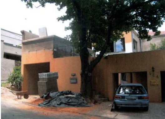
The house Anne and David are building
