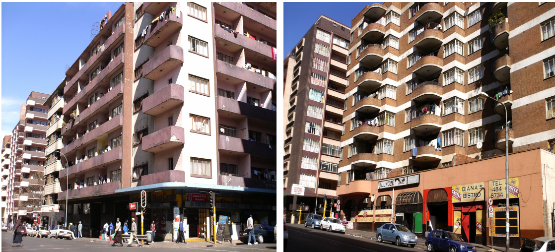
Photos 7 and 8: Some derelict buildings in Doornfontein (left) and Hillbrow (right). Overcrowding, illegal activities and non-compliance to by-laws is common in these buildings. Evicting illegal occupant is often a major challenge.
