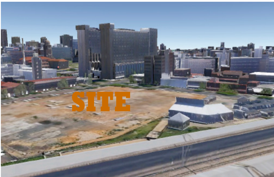
FIG 79- Ariel View of Site
