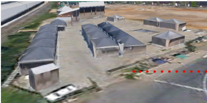
FIG 86- Train Station entrance
