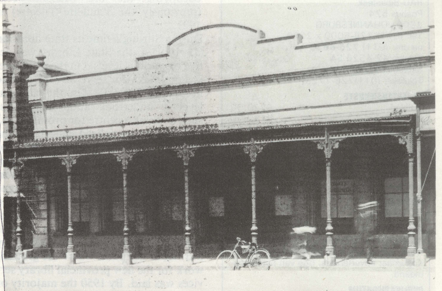
The Frank Stevens building, 233 Church Street, where the State Library was housed from 1903-1920.
