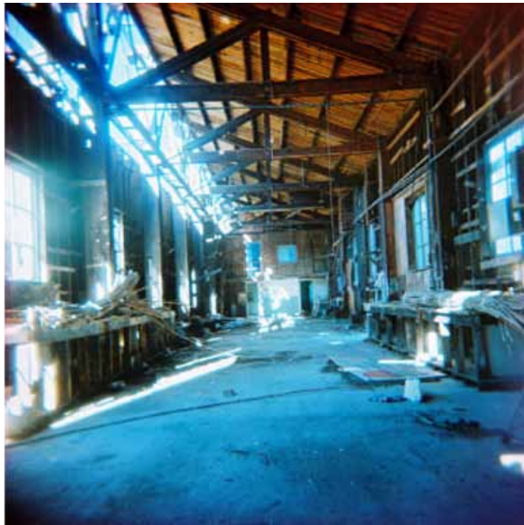
Figure 4 Interior of Shipwright Building
