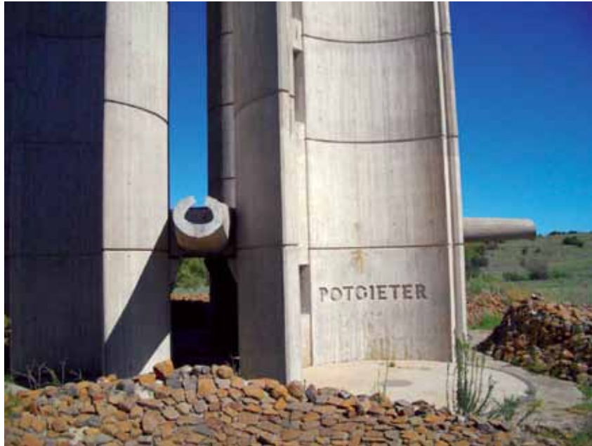
Figure 9 Spouts emerging like cannons through the intercolumniations to discharge into the surrounding rubble-lined bowls.
