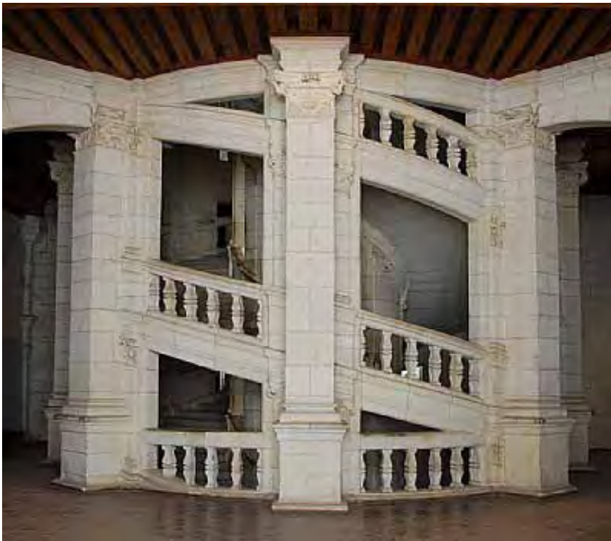
Figure 11 Attributed to Leonardo da Vinci, double helix staircase, Château de Chambord, 1519-47 (photograph: the author).
