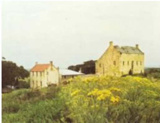
Figure 5: Lombard's Post, buildings and walls forming a hexagonal farmyard. 23
