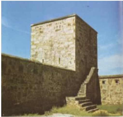
Figure 6: Fort Brown, the gun tower from the parade grounds 27
