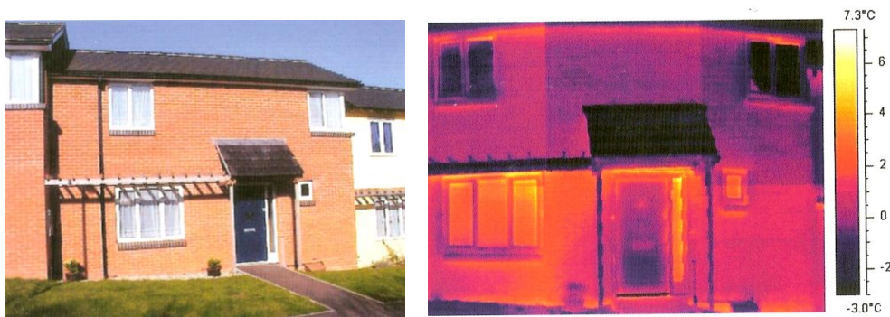
Figure 2: Masonry house and thermo graphic image of masonry house. (Allin 2005:54)
