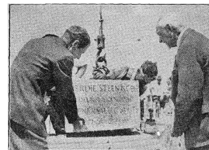
PRETORIA UNIVERSITY LIBRARY. General Smuts this morning laid the foundation stone of the new library at Pretoria University. On the left is Mr G. Moerdijk, the chairman of the University Council.
