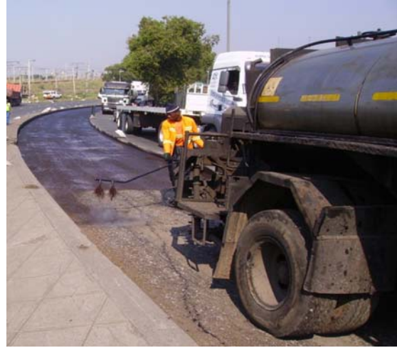
Figure 7: Tack coat application
