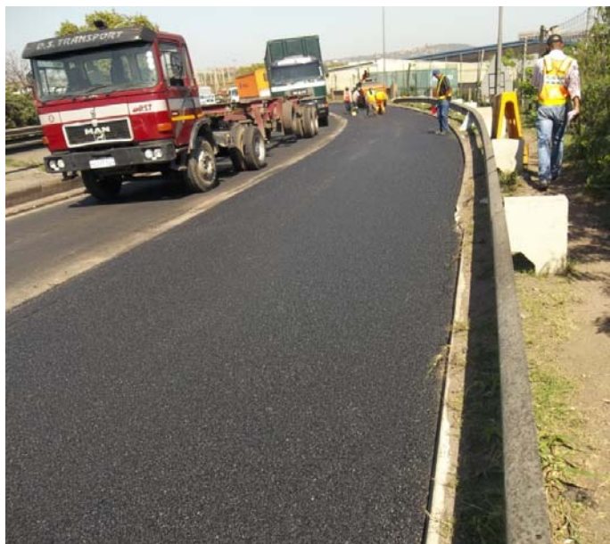
Figure 8: Finished surface of HiMA layers
