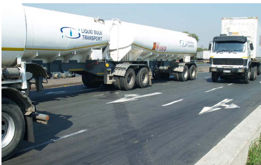
Figure 9: Finished surface of the road after SMA surfacing
