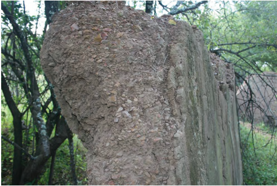
Figure 3 Profile of a rammed earth wall on the farm Zeekoegat (source: photograph by the author).
