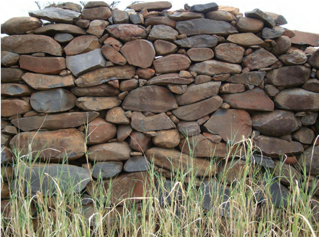
Figure 3 Part of the stonewalling at Molokwane (photograph: the author).
