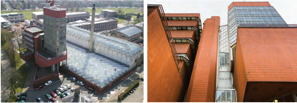
Figure 9 Engineering Building (1959-1963), Leicester University by Stirling & Gowan (Google images).
