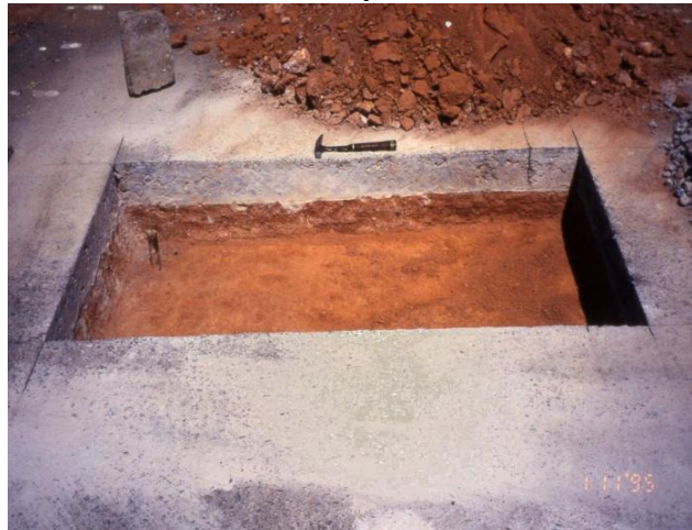
Photo 6: G1 layer cut like concrete.
