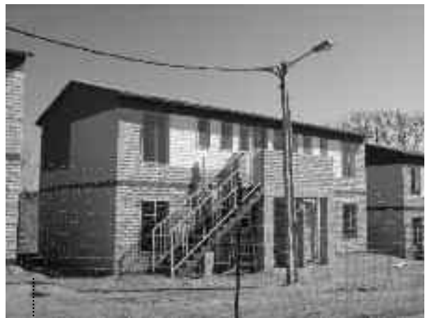
Figure 1. Semi-detached low-income (RDP) units on two levels in Pennyville.
