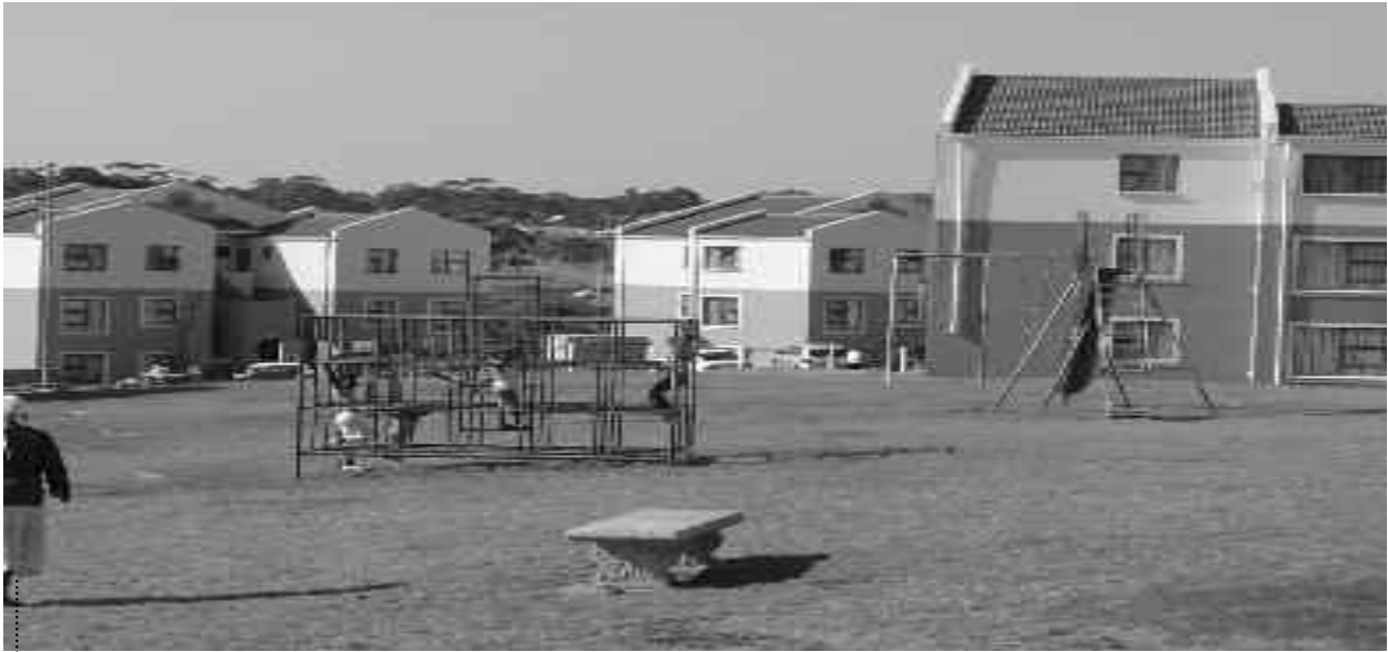
Figure 2. Different building types and unit sizes organised around communal play space in Amalinda.
