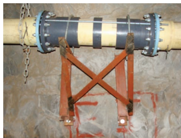
Figure 5—Expansion joint installation
