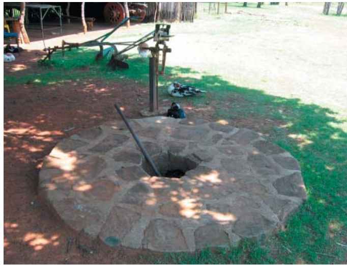
Figure 1 Circular paved stone area where a hot iron tire is placed over the wooden rim of a wagon wheel (photograph: M. Naudé).
