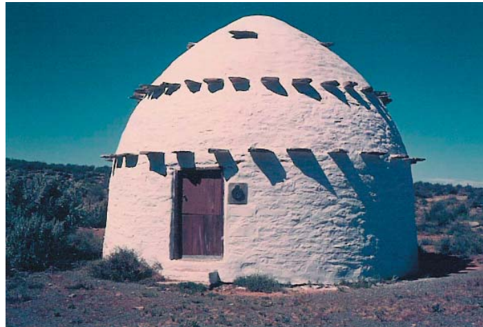
Figure 28 Corbelled dwelling in Namakwaland (photograph: Ditsong: National Museum of Cultural History, Pretoria).
