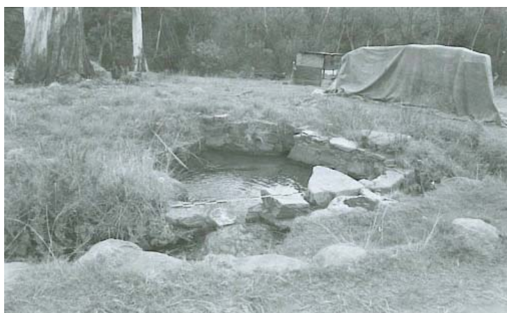
Figure 12 Circular ‘distributor’ dam where water from the principal water furrow is distributed into several secondary furrows – Lydenburg district, Mpumalanga Province (photograph: M. Naudé).
