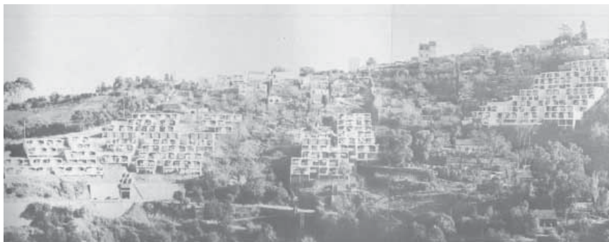
Figure 41 Roland Simounet’s housing project in Algeria, 1959 (source: Zeynep 1997: 164).
