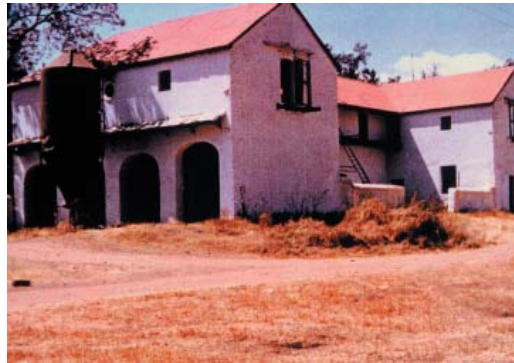
Figure 18 Horse stables and cart shed on the farm Zwartkoppies (Pretoria) erected ca. 1886 (photograph: M. Naudé).
