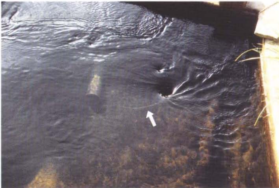
FIG. 1 Typical vortex in a header box showing air entrainment (arrow) into a pipe
