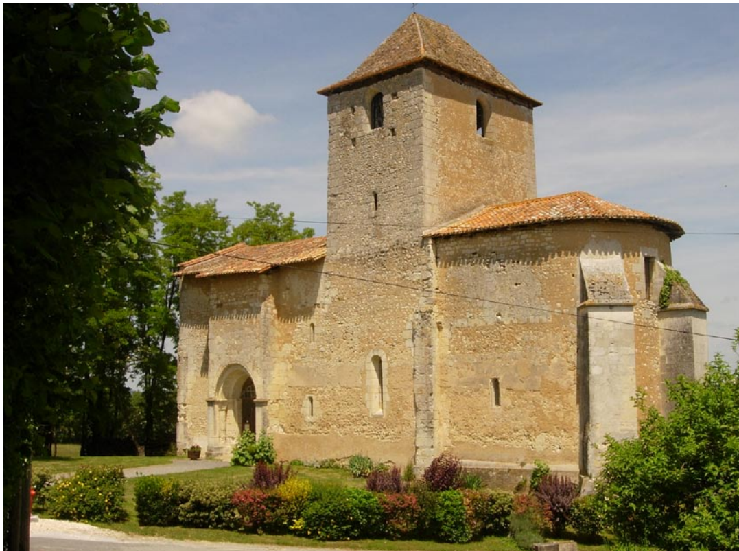
Figure 1 The church of Notre-Dame de Bourg-du-Bost with its sparsely decorated rounded Roman arch side-entrance (photo: Alain de La Ville).
