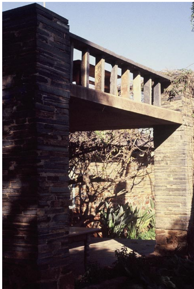
Figure 11 Railing (long bar of slate) on top of the porte-cochere along the front (northern) façade of the Preller dwelling (photograph: M. Naudé).
