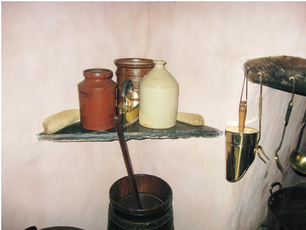
Figure 10 Triangular slab of slate mounted in the corner of the kitchen and used as an open shelf directly adjacent to the hearth, dwelling at the Pioneer Museum, Silverton (photograph: M. Naudé).
