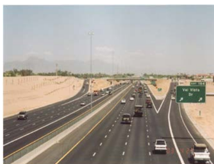
Figure 5. Superstition Freeway in 2003 with ARFC surface (Courtesy of Arizona DOT)
