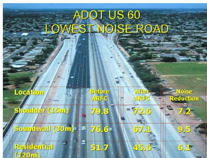
Figure 6. Superstition Freeway 2002 noise reduction due to asphalt-rubber open graded mix, courtesy Rubber Pavements Association, noise measured in dBA
