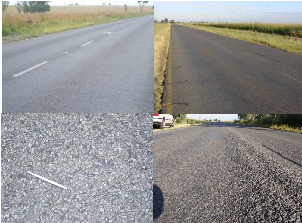
Photograph 5: Road P5-1 to the east of Springs within Gauteng
