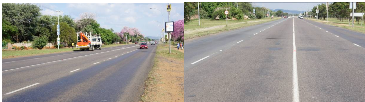
Photograph 3: Thabo Mbeki Road (P1-5) through Mokopane (Potgietersrus)
