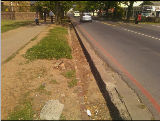
Figure 15: Gutter on side of road along Bird Street
