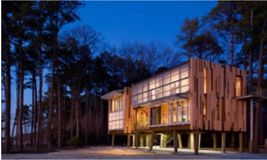
Figure 2: Loblolly House; Maryland; USA
