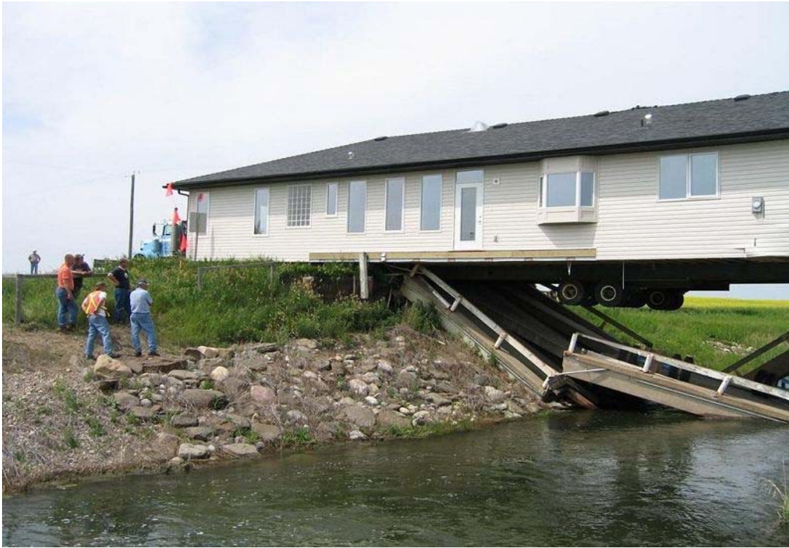
Figure 3 Poor site conditions planning of a modular house 1c
