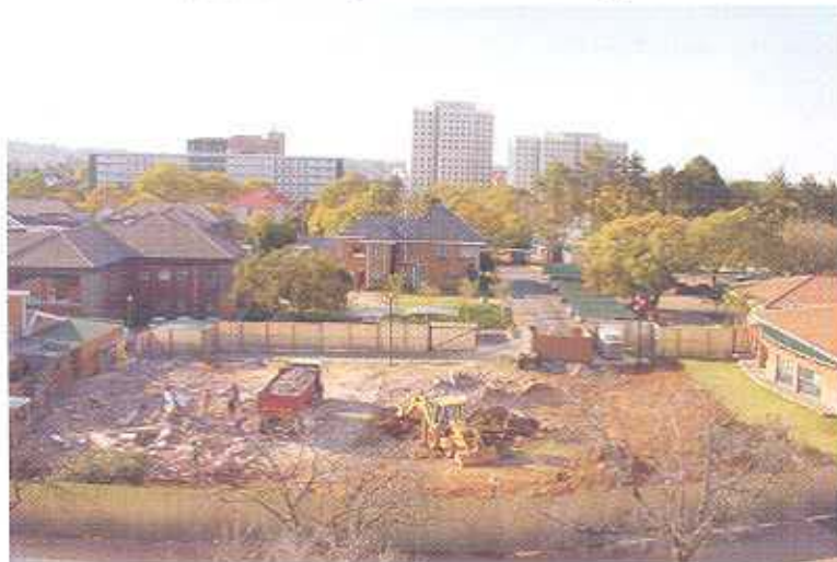
October 2002, clearing the site
