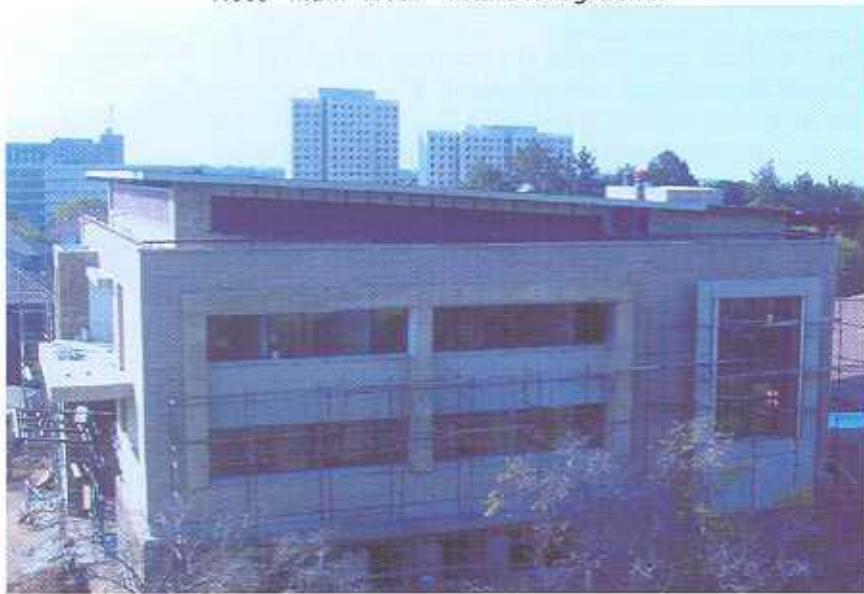
June 2003, building is almost completed
