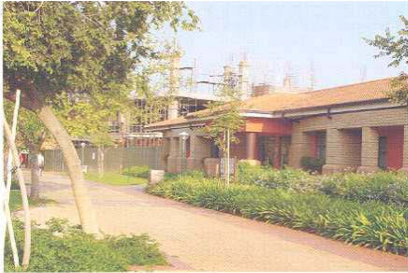
January 2003, second floor up and the start of the third floor. Note "main' FBI" in the foreground.
