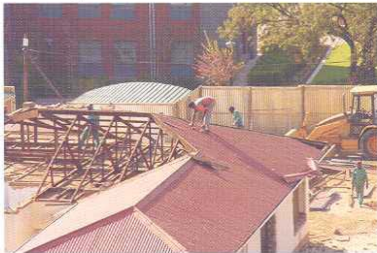
October 2002, the demolition begins!
