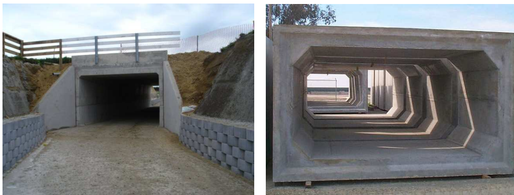
Figure 2.3.1: Photograph of portal and rectangular culverts, (Entranceways, 2010; Midstate Precast, 2010).
