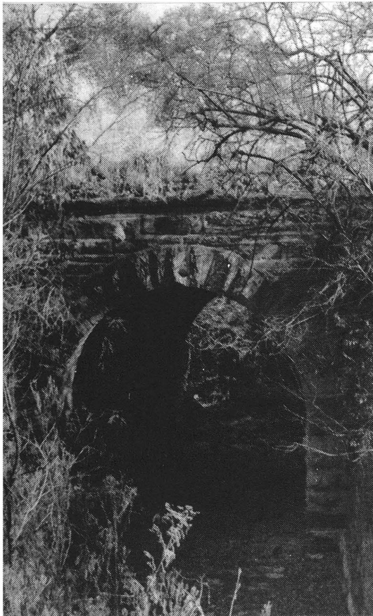
Old arched culvert under the previous NZASM railway near Fountains Valley entrance Photo: R.C. de Jong
