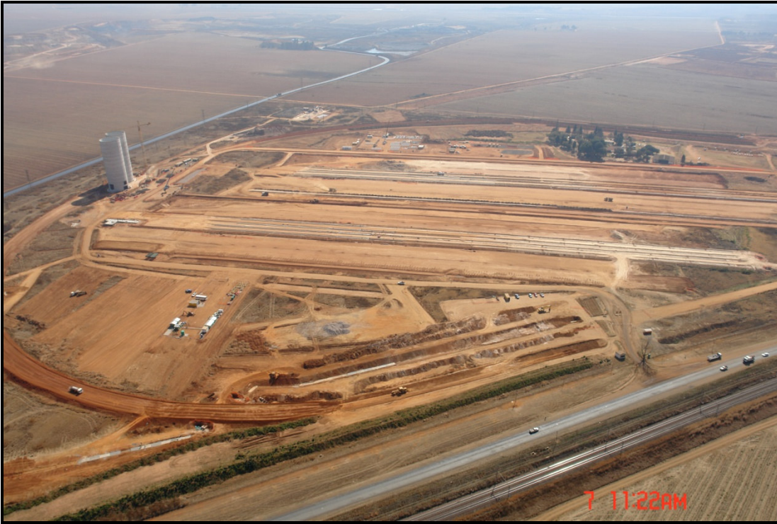
Figure 5: An aerial view of the new construction site
