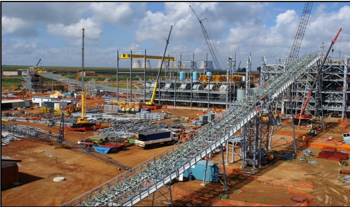
Figure 8: A new conveyor belt being constructed
