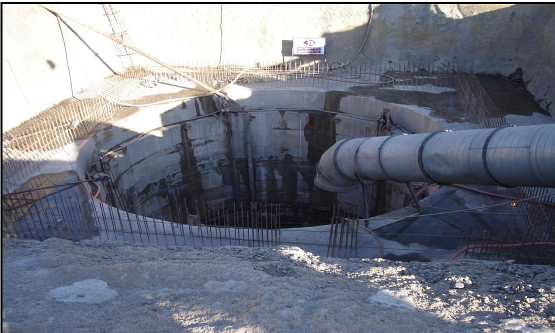
Figure 6: A vertical shaft being constructed out of concrete (Rossouw 2008: Zondagsfontein Colliery)
