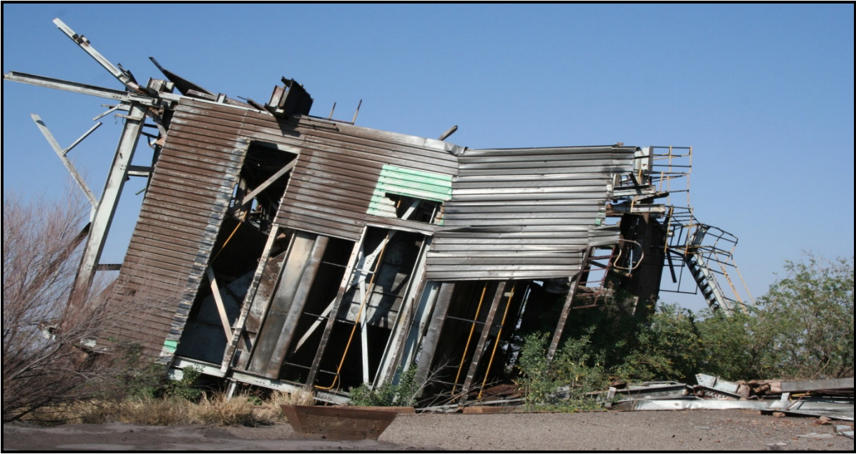
Figure 13: Steel structures being broken down into manageable sizes
