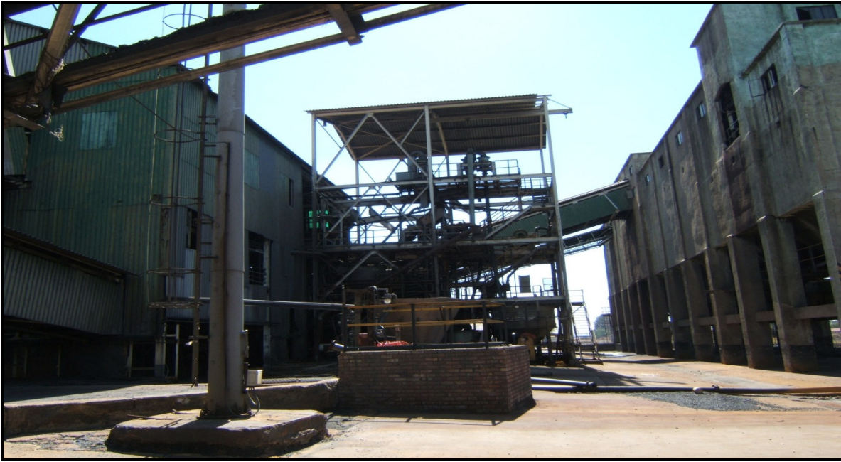
Figure 11: The infrastructure on an active coal mine
