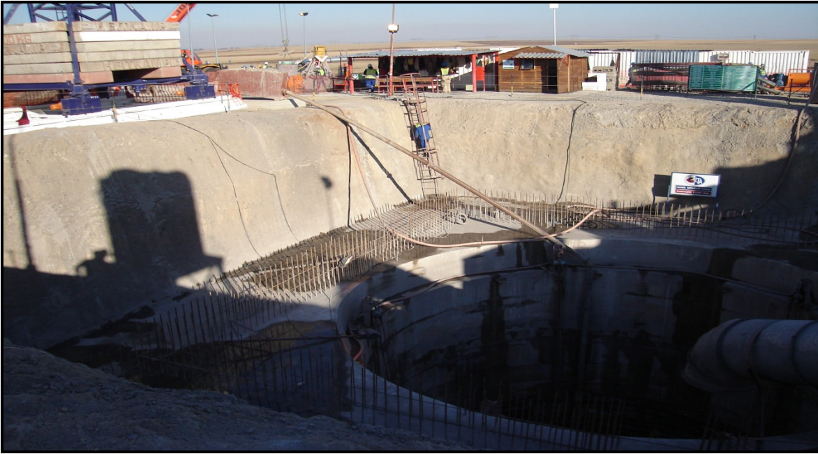
Figure 7: Temporary retaining walls around the new shaft
