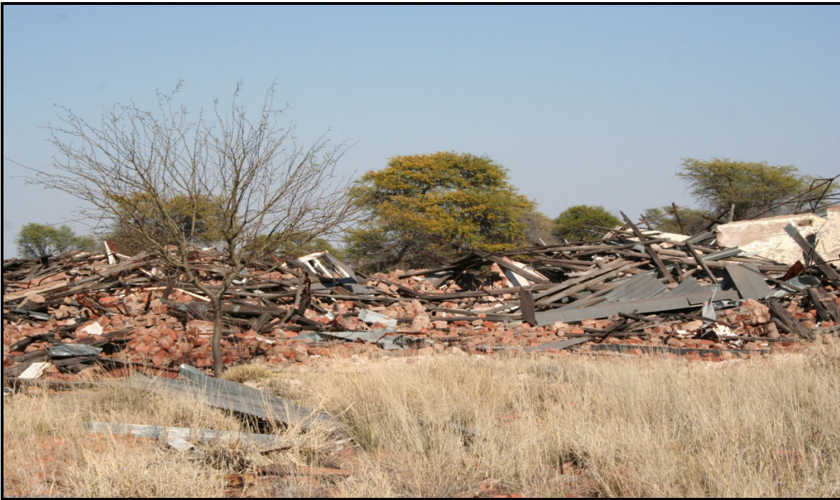
Figure 12: Infrastructure being demolished after coal mine closure
