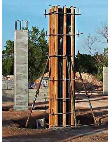
Figure 11: Concrete column and formwork. (Source: www.builderbill-diy-help.com )
