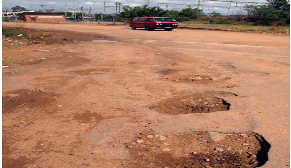
Figure 14, Taryn Eliot, Training for Township Initiative, 2007, illustrates the poor condition of some of the roads
