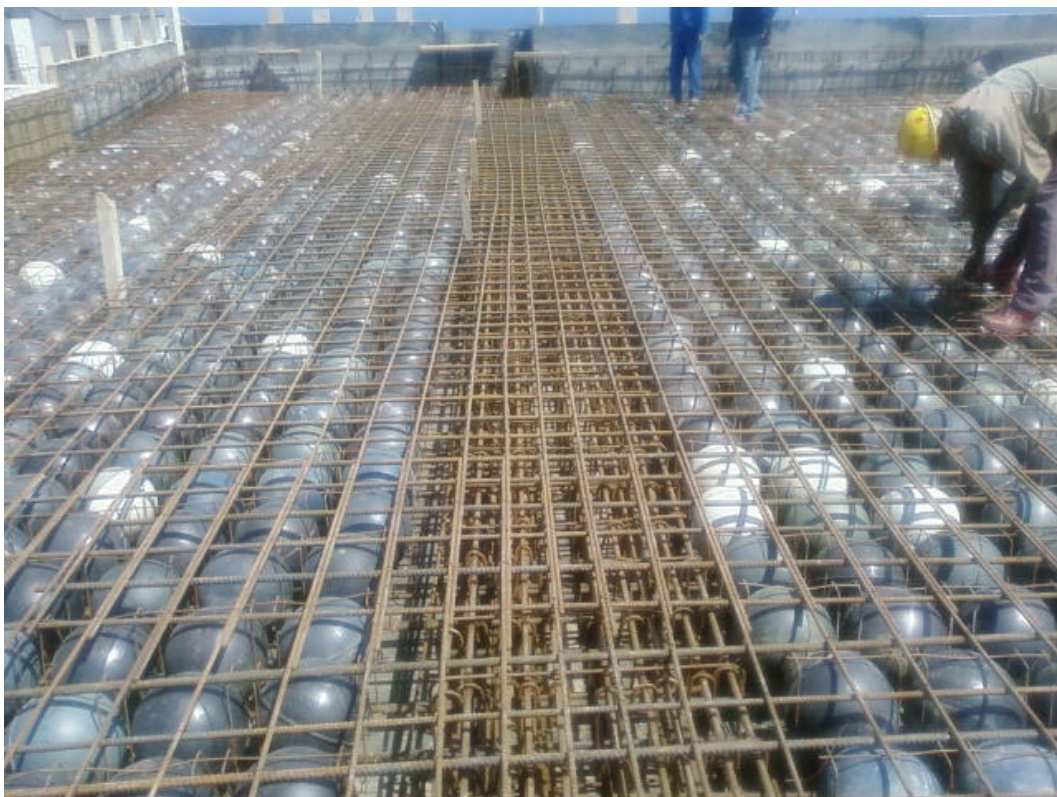
Figure 14: Cobiax slab ready for concrete to be poured (own information)
