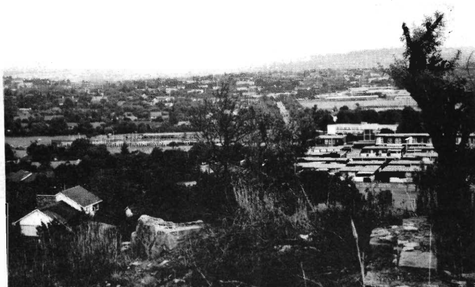
The South-East Pill-Box as it looked in September 1972 and as it looks today. (As viewed from the east side).
