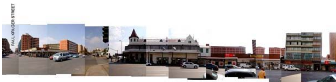
Panoramic view on Paul Kruger Street, West elevation
