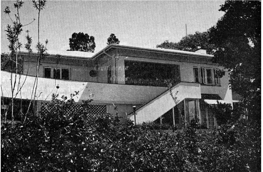
„Bergloo”, St. Patrickweg 251, Muckleneuk, Pretoria. Woning van dr. Willem Punt waar die Genootskap Oud-Pretoria in 1948 gestig is. „Bergloo”, 251 St. Patrick Road, Muckleneuk, Pretoria. Residence of Dr. Willem Punt where the Old Pretoria Society was founded in 1948.
