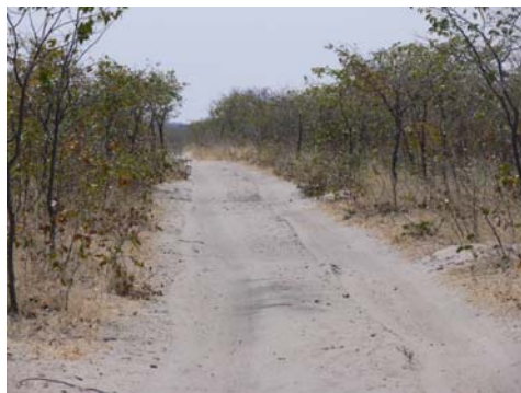
Photograph 1: Typical sand track prior to upgrading
