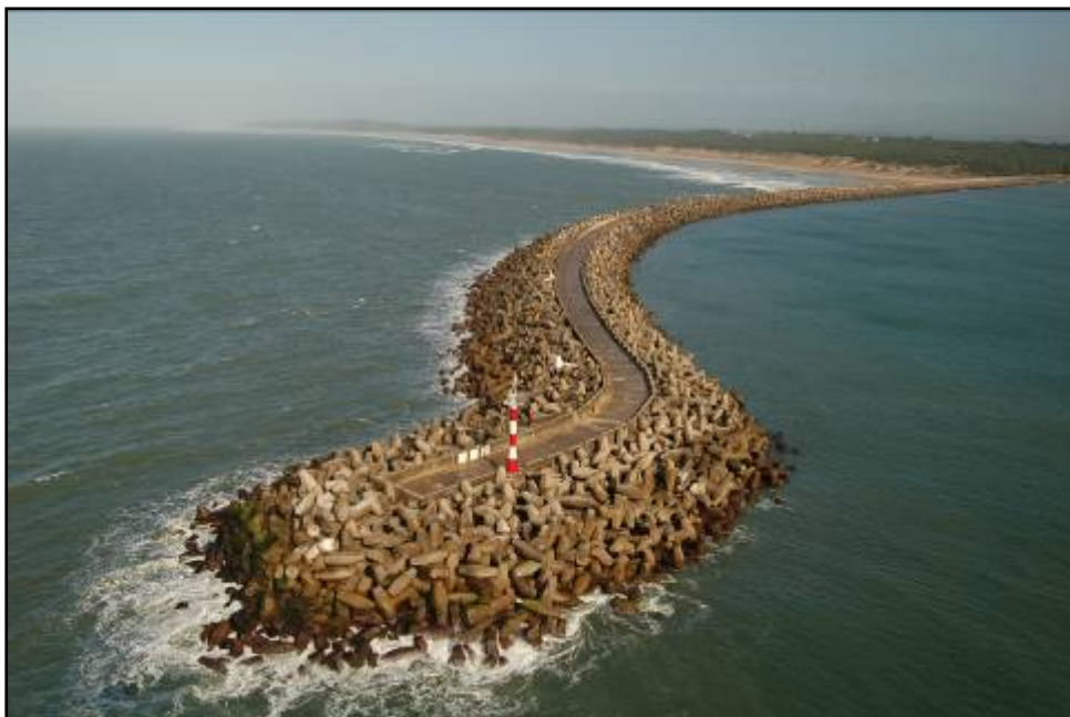
Figure 6: South Breakwater at the Port of Richards Bay
