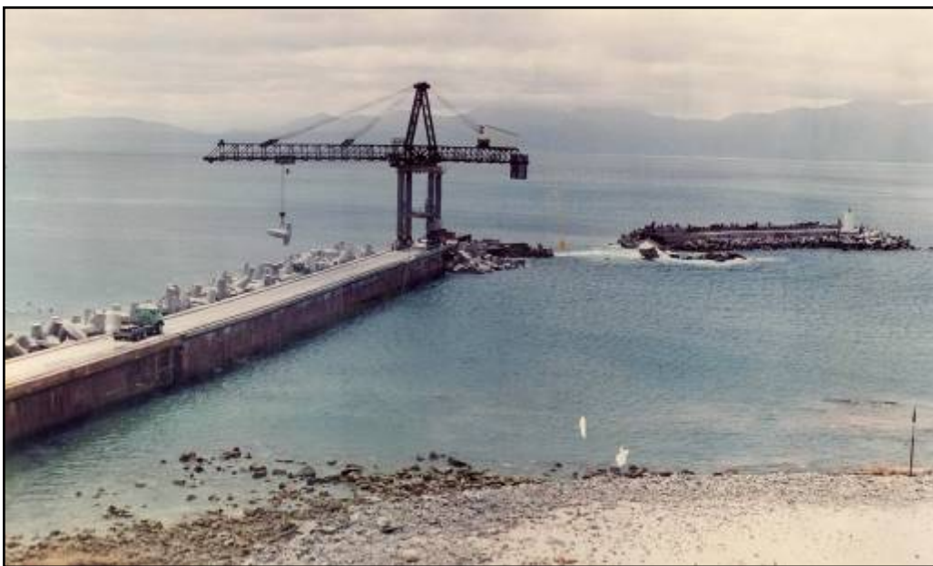
Figure 10: Breakwater Failure due to Focusing of Storm Waves
