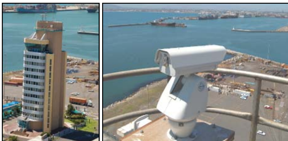
Figure 1. Video Camera on top of the Cape Town Port Control Building
