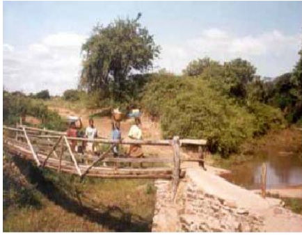
Fig. 1: Footbridge linking a village and fields
