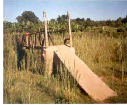
Fig. 2: Footbridge linking 2 villages
