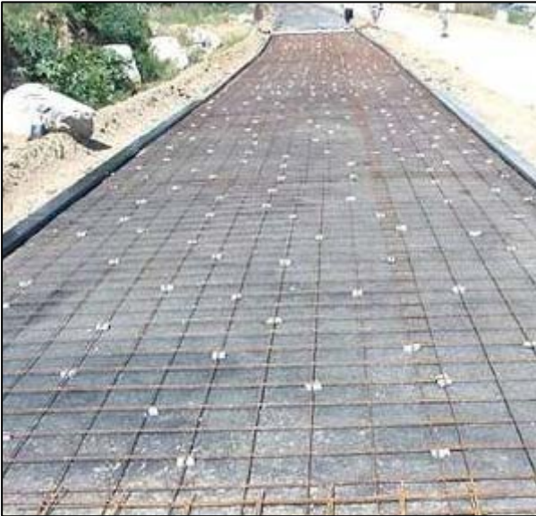
Photo 1: View along CSIR section prior to casting concrete
