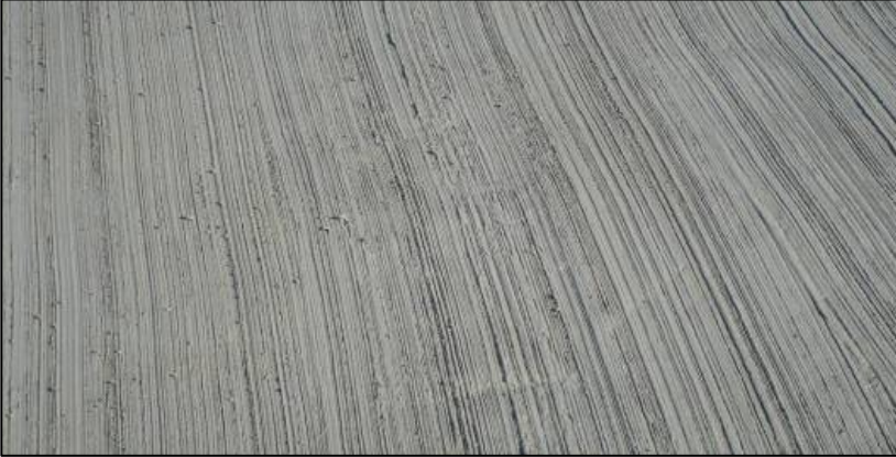
Photo 10: Hand floating prior to brooming (note the use of a bridge)
