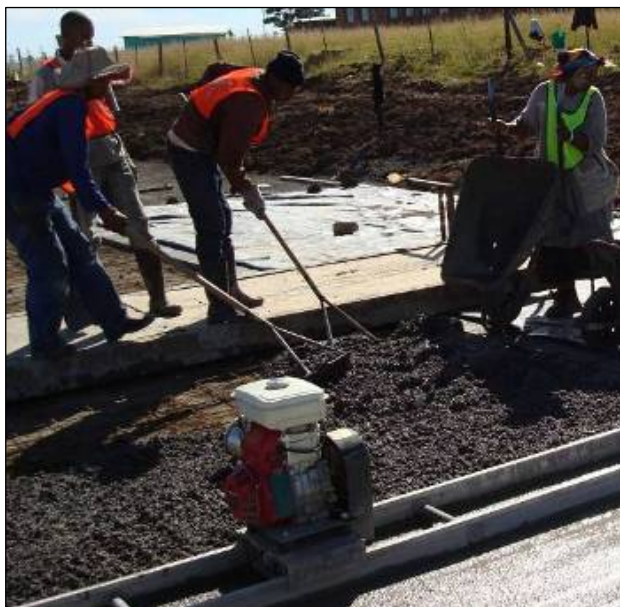
Photo 6: Use of bridge during concreting operation
