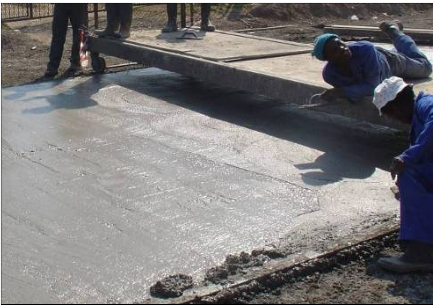
Photo 10: Hand floating prior to brooming (note the use of a bridge)
