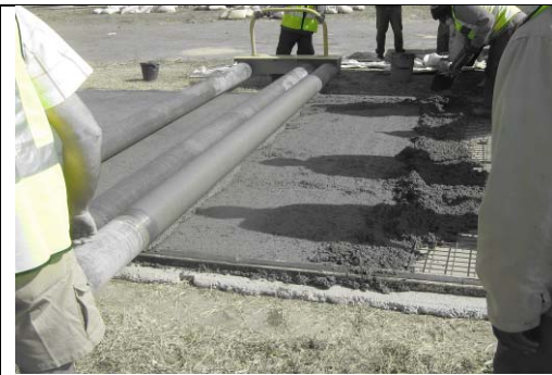
Figure 5: Oscillating triple roller screed in action
