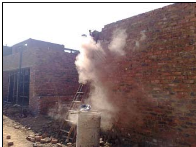
Figure 21 - Labour Chasing Channels (own information)
