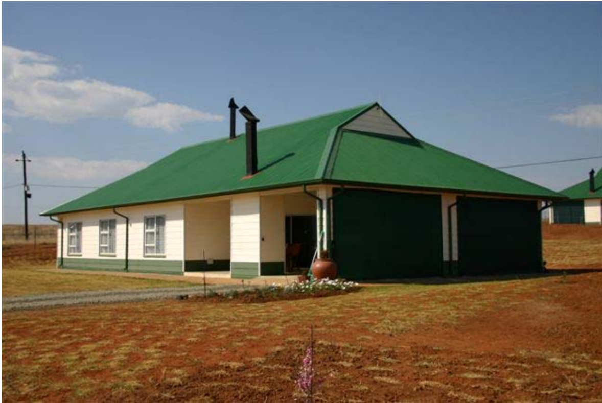
Figure 14 - Completed LWFS unit (Own information)
