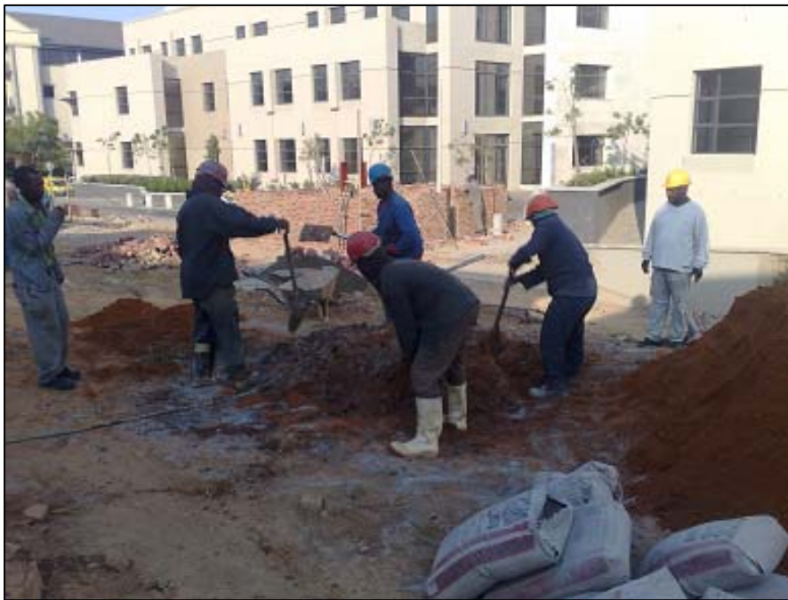
Figure 19 - Labourers mixing dagga (Own information)
