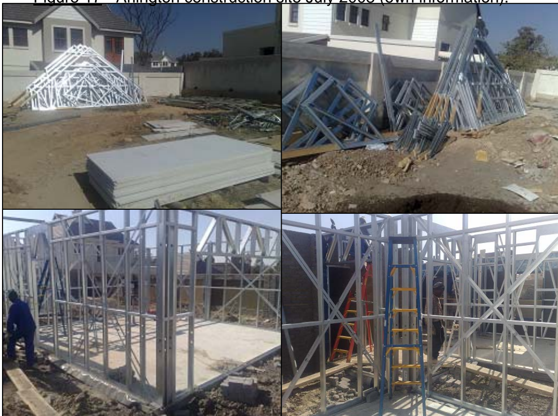
Figure 17 - Arlington construction site July 2008 (own information).
