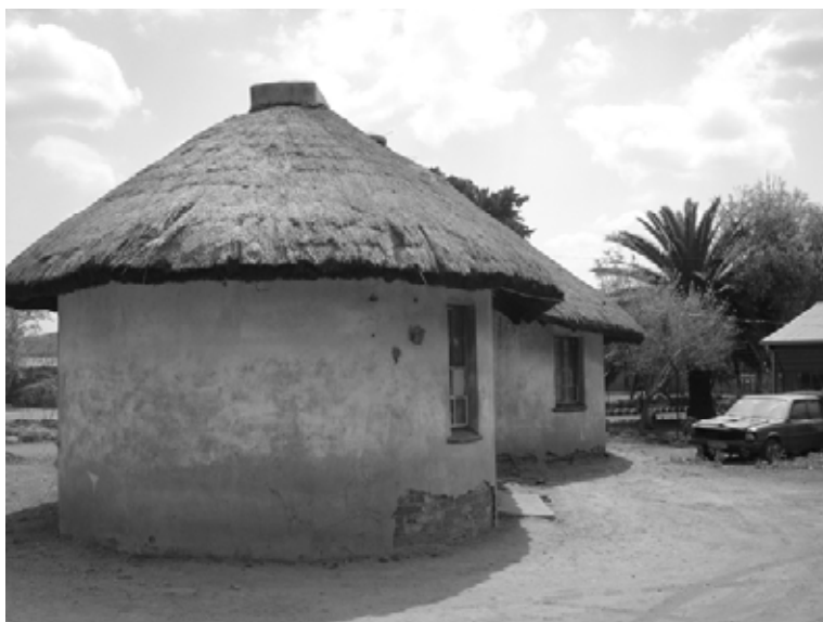
Figure 8 A surviving rondavel in Mamelodi, built in 1947 (Photo: G Steyn)
